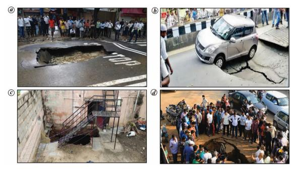
Figure 1. Cavity formation incidents due to (a) water pipe burst (26 June 2018, Mumbai); (b) metro tunnelling (2 August 2016, Bengaluru); (c) metro tunnelling (1 October 2021, Bengaluru), (d) improper compaction of subgrade (5 November 2016, Hyderabad).
